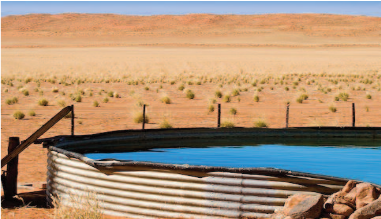
Water butts collect and store rainwater
